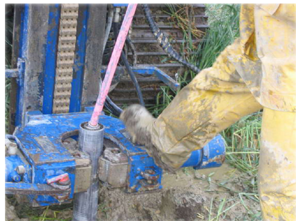
Fig. 11 Installation of temperature sensor through high-pressure channel of drilling rod
